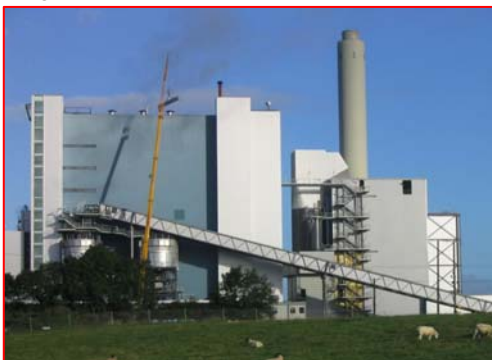
Fig. 3 Desulphurization and Dedust Island of Lanesborough Power Plant in Ireland
