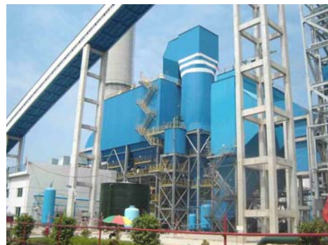
Fig. 6 Desulphurization and Dedust Island of Power Utility Division, Sinopec Guangzhou Co., Ltd.
