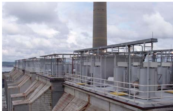
Fig. 11 Roof Elevation of Units 1-6 after Project Completion
