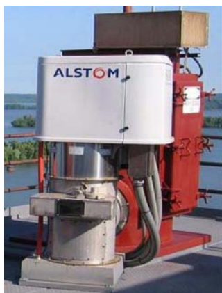
Fig. 5 SIR supply rated 70 kV, 800 mA or 60 kV 1000 mA (identical exterior)
