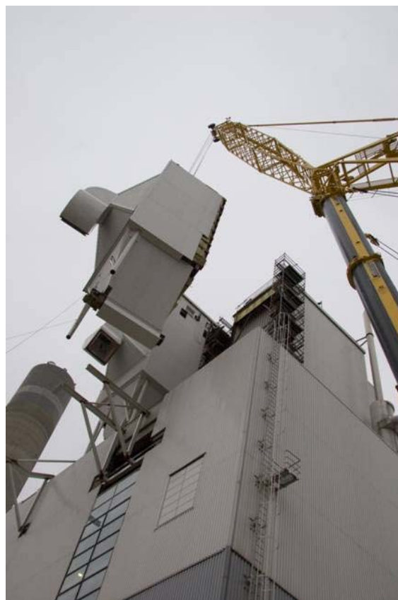
Fig. 4 Heavy lift of the second ESP field
