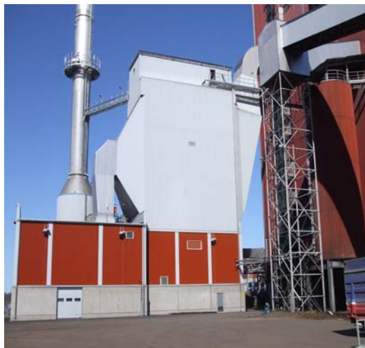
Fig. 8 ESP after FBC in Heinola, FI
