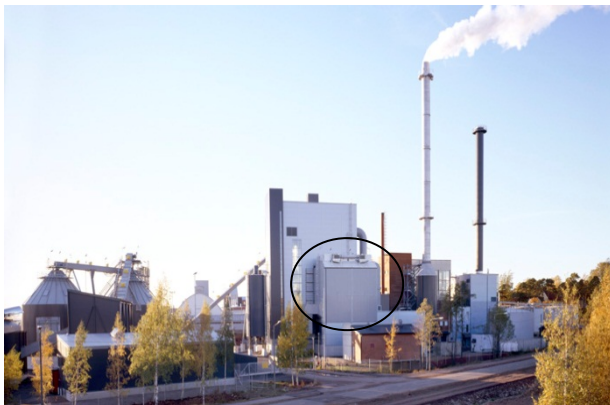
Fig. 4-1: Ion Blast ESP in a biomass power plant
