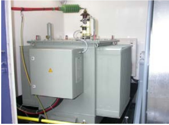
Fig. 3: Integrated 500Hz HV transformer
