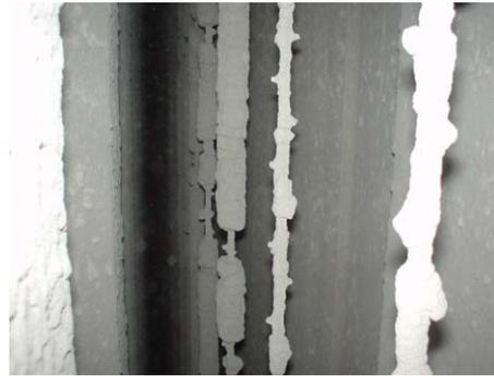
Fig. 7-2: Figure not cleaned discharge electrode
