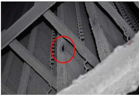
Fig. 7-1: Discharge frame misalignment with local flash-over marks
