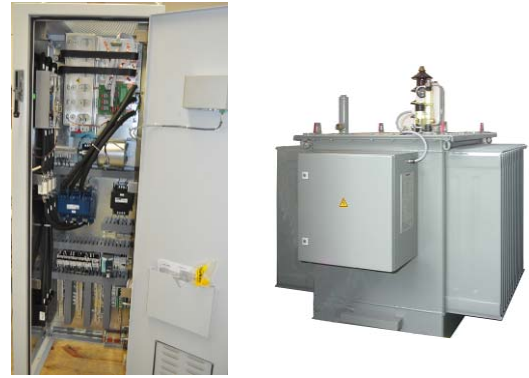
Fig. 3-5: SIPREC I control cubicle and HV transformer rectifier (2011)
