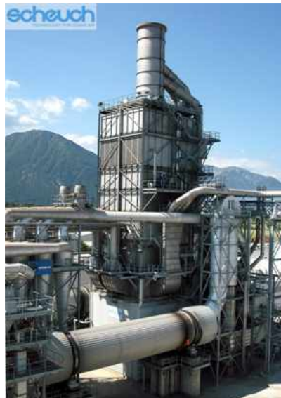
WESP with condensing system
