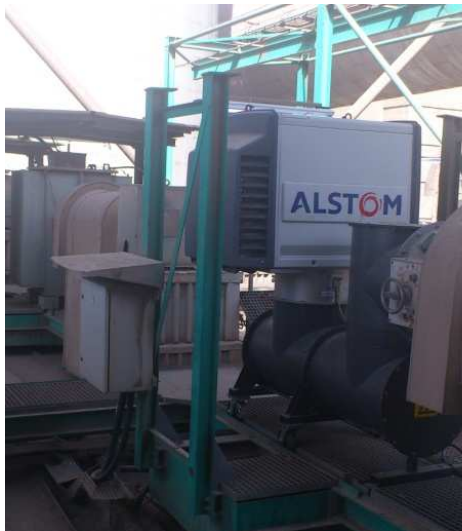
Fig. 2.3. Installation of SIR
