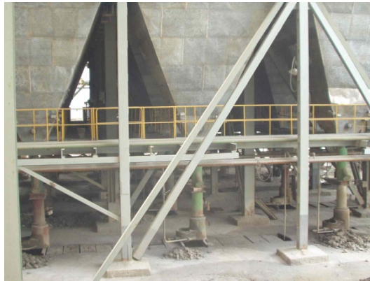
Figure 1: ESP Fly Ash Hoppers
