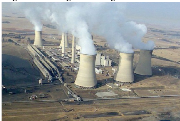
Figure 19. Arnot Power Station, 6 x 350 MWe, South Africa. HRFFs on Unit 1 – 3. ESP to HRFF retrofit.
