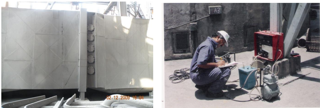
Fig.4: Sampling ports and Emission Monitoring
