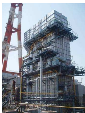
Figure 13 Vertical Flow Type WESP in Japan
