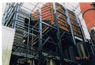
Figure 10 WESP for Oil-Fired Boiler in Austria
